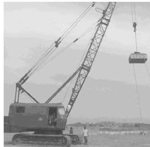
Fig. 4: Dynamic Compaction in Progress on Site
